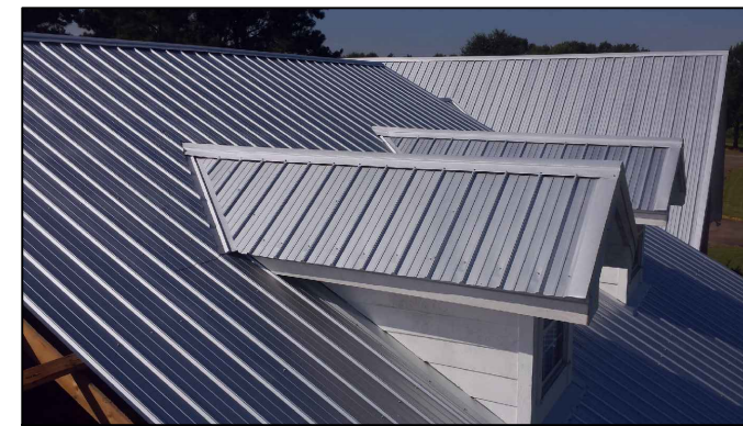
STANDING SEAM ROOF ROOF MATERIAL
