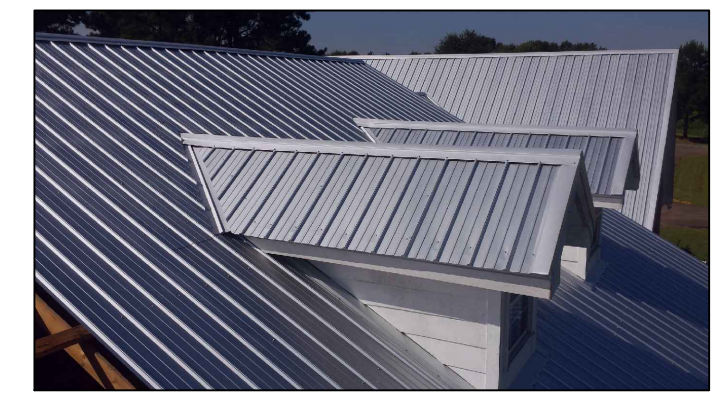
STANDING SEAM ROOF ROOF MATERIAL
