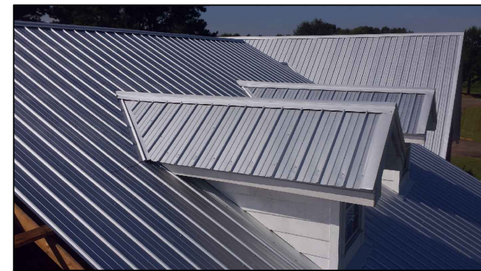
STANDING SEAM ROOF ROOF MATERIAL
