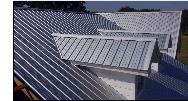
STANDING SEAM ROOF ROOF MATERIAL
