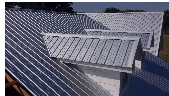
STANDING SEAM ROOF ROOF MATERIAL
